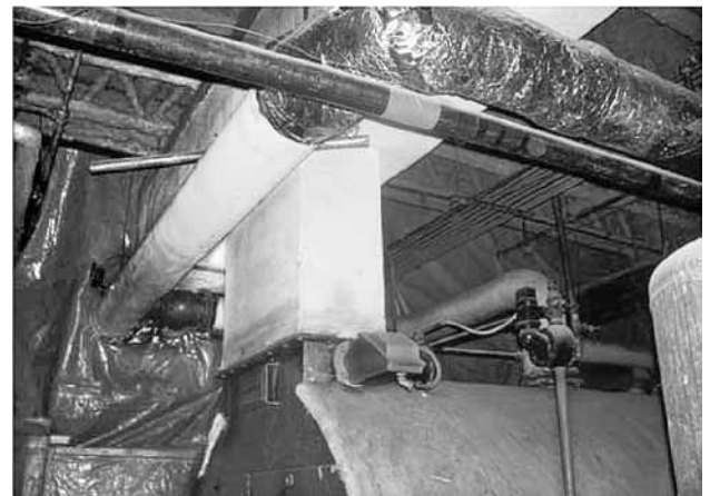
Figure 45: Boiler Insulation Containing Asbestos
