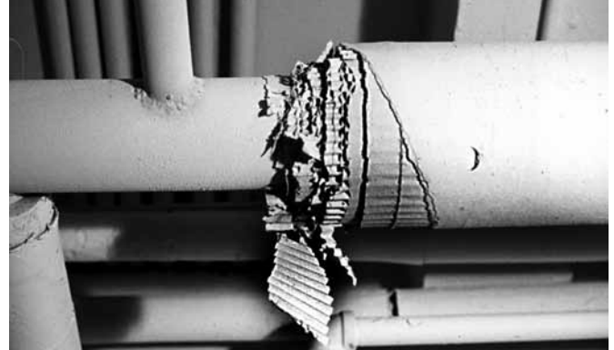
Figure 44: Air-Cell Insulation Commonly Used Around Pipes
