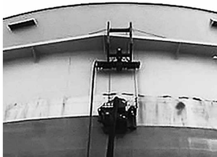
Figure 21: Wind Girder Scaffolding
